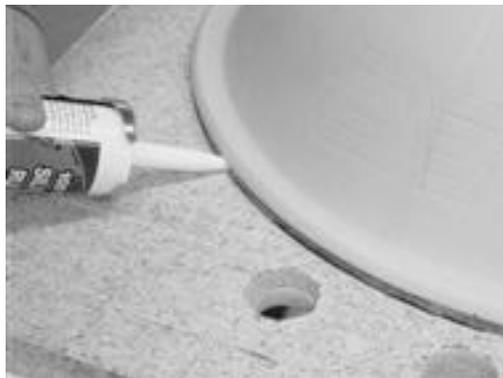
Install a bead thick enough to fill the area between the quartz top and the bowl's lip.
