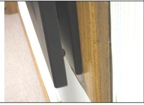
3. Place the nose of your pliers into the hinge cup of the middle hinge and allow the flat side of the pliers to rest on the screw of the hinge plate that is attached to the frame of the cabinet as shown in the picture.
