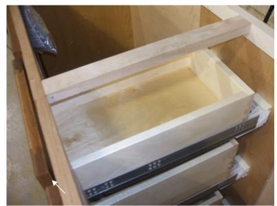
To align the drawer front to be flush against the cabinet Drawer fronts have bumpers placed on back edge that will prevent drawer from laying flat against the frame.
