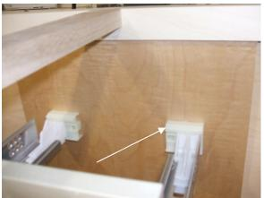
This shows the drawer plugs back in alignment after drawer was pulled out and properly re-aligned.
