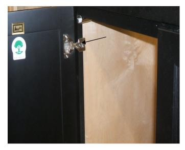
To adjust the door up, loosen the center screw on both hinges but DO NOT remove, move the door to the desired position and retighten this screw on both hinges. To adjust the door down, loosen the center screw on both hinges but DO NOT remove, move the door to the desired position and retighten this screw on both hinges.
