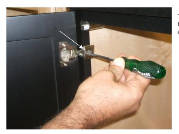
To adjust the door closer to center of cabinet turn the front screw clock wise. To adjust the door out from the center of the cabinet turn the screw counter clock wise.
