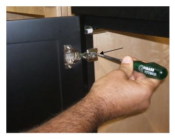
To adjust the door closer to face of cabinet turn the back screw clock wise. To adjust the door out from the face turn the screw counter clock wise.
